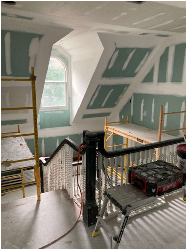
Stairway Landing (Rm 300)
