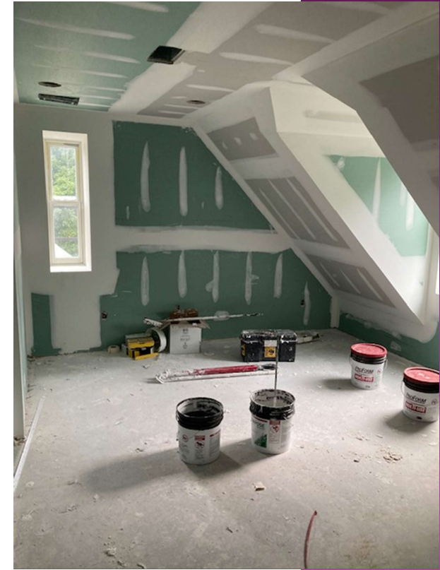
Back Right "Attic" (Rm 305)
