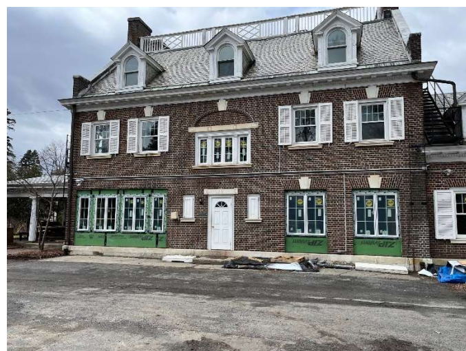
Back of house in April with new windows installed
