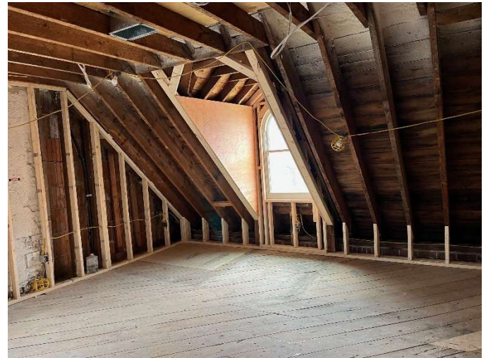
Front Left Third floor (Room 302) in April
