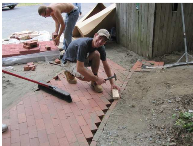
Redoing the sidewalk to complete the restoration of the Garage
